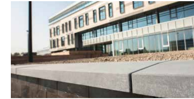
The two sealant-free coping stones are close-fitting, thus eliminating the need to seal any expansion joint.
